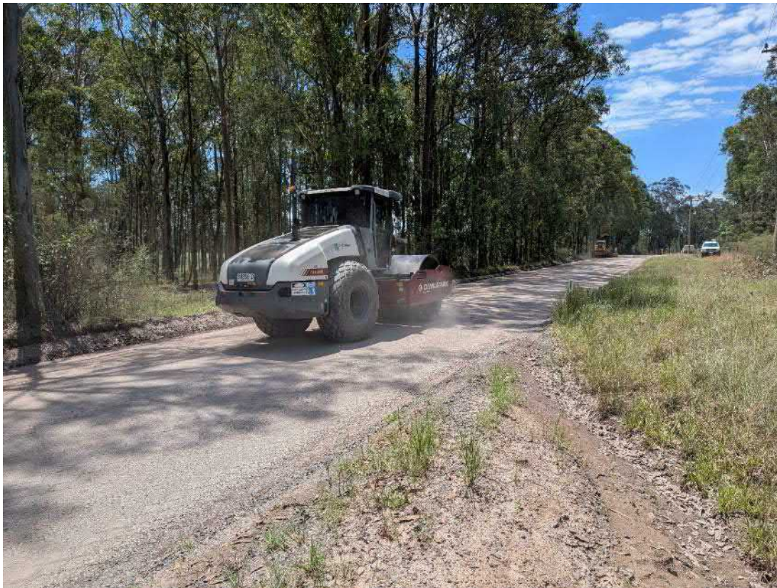
Plate 3.1: Grading and rolling of East Seaham Road within the study area.
