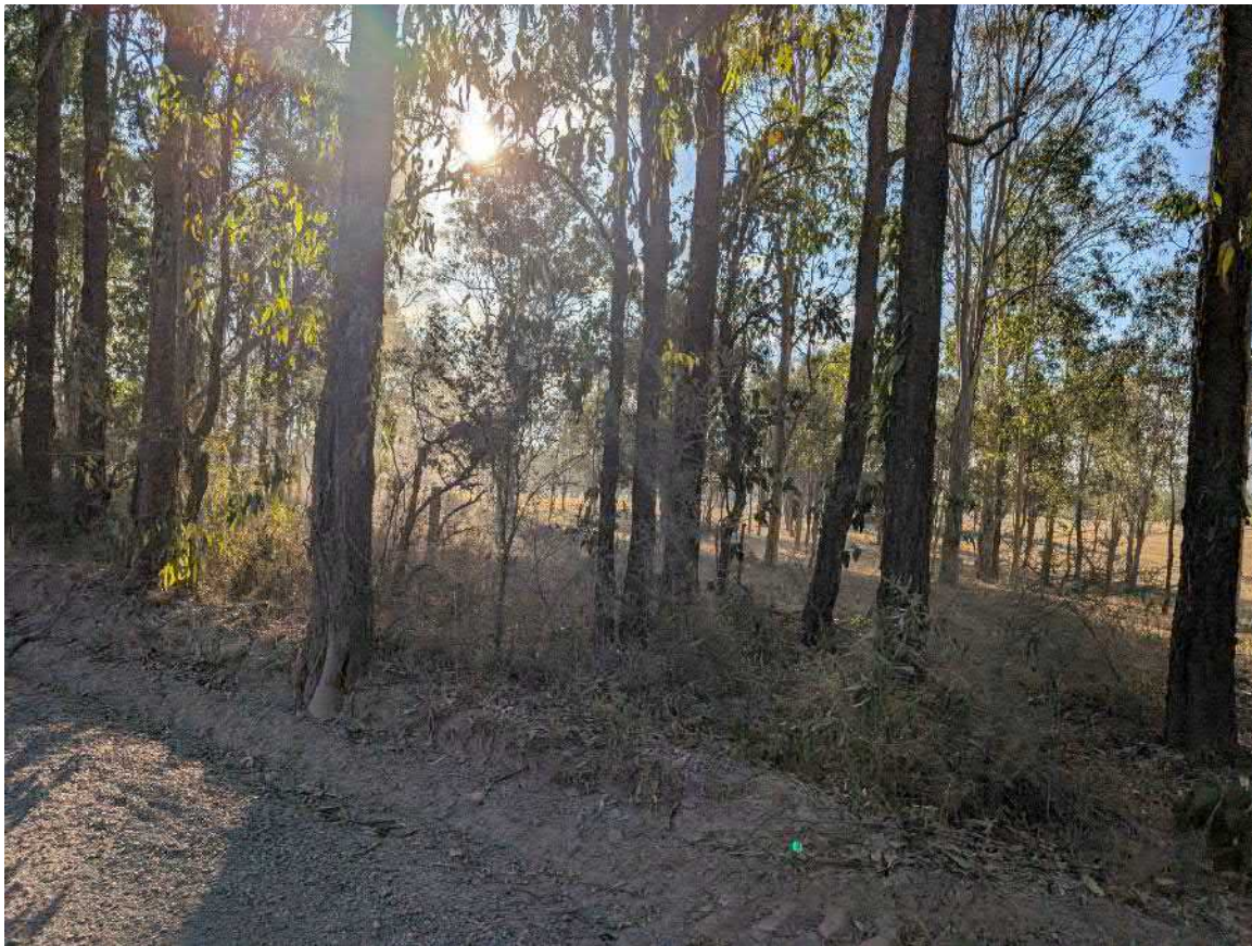
Plate 3.2: Erosion, gravel incursion and dust from continued gravel road maintenance.
